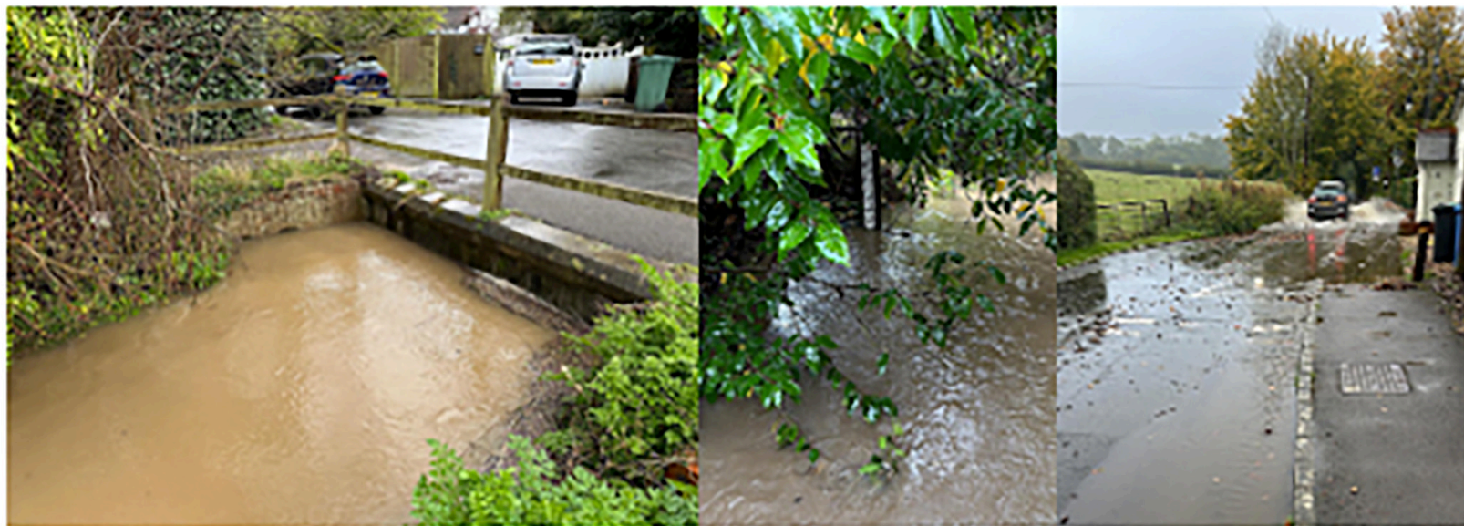
FLOODING - Residents at the east end of the village have to keep an eye on river levels and flood warnings
